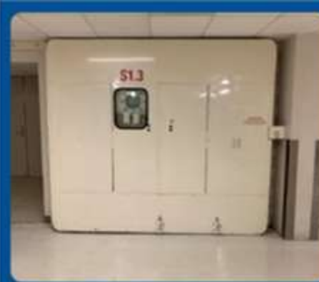
Watertight enclosure to prevent floodwater damage
